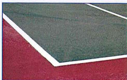
RiteWay Crack Repair System: Finished repair.
